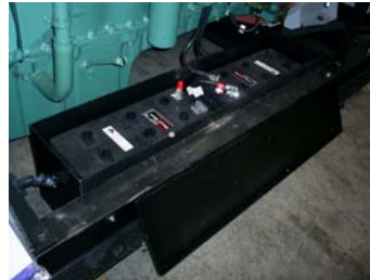
Battery box and batteries are mounted inside the main frame rails with the cutoff switch mounted on the pedestal and below the control panel.
