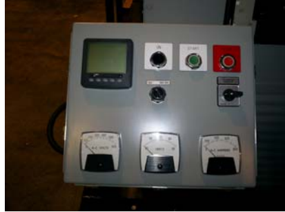
Control panel and gauges for both the generator and the engine. The main breakers are installed in the generator with easy access for connections.
