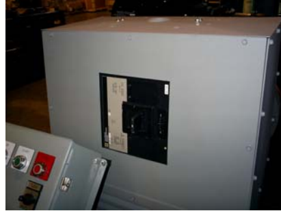
Control panel and gauges for both the generator and the engine. The main breakers are installed in the generator with easy access for connections.
